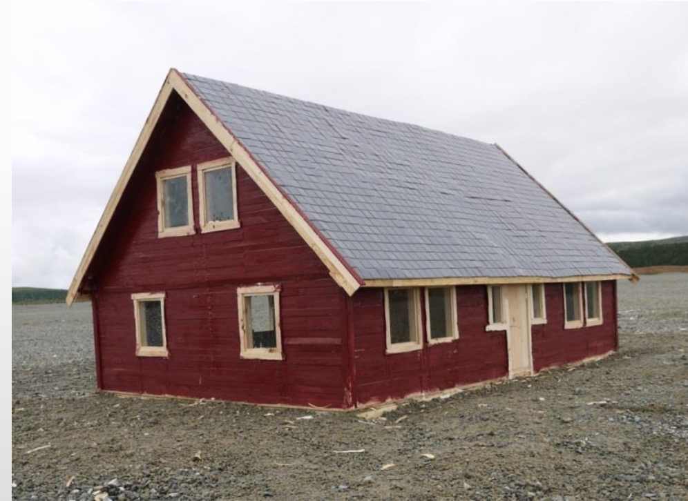
Figure 14: Photo of the ES before the explosion
